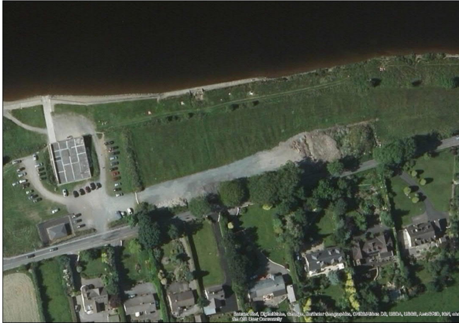
Photograph 7 Overview of the Proposed location of the extension to Knockieran Car Park.
