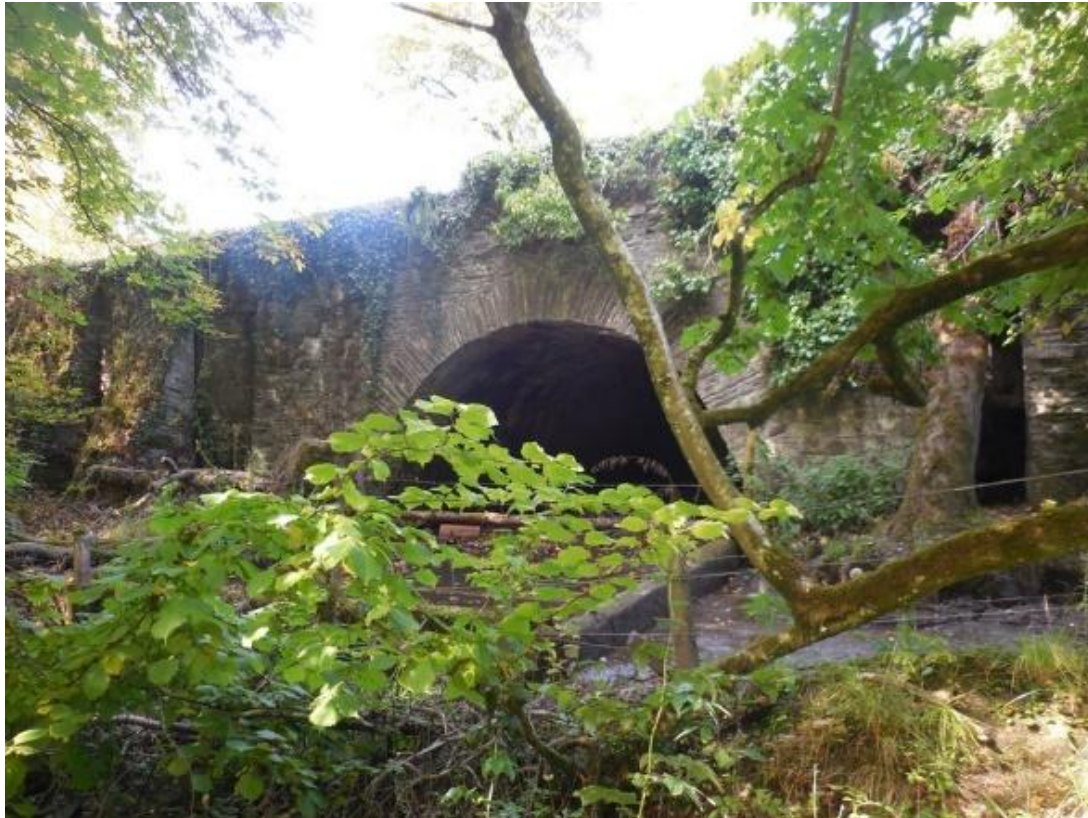
Plate 5 Looking north to unnamed bridge Russborough.
